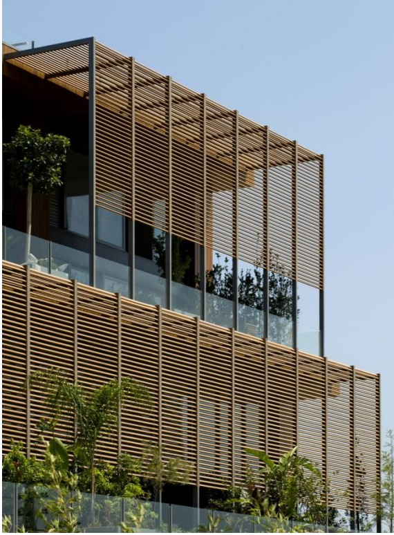
Şekil 2.5. Güneş kırıcı elemanların kullanımı – 7800 Çeşme Residence & Hotel ( https://www.archdaily.com/161768/7800-cesme-residences-and-hotel-emre-arolat-architects/50155f9528ba0d02f0000fe7-7800-cesme-residences-and-hotel-emre-arolat-architects-image/ ) (20.09.2019)
