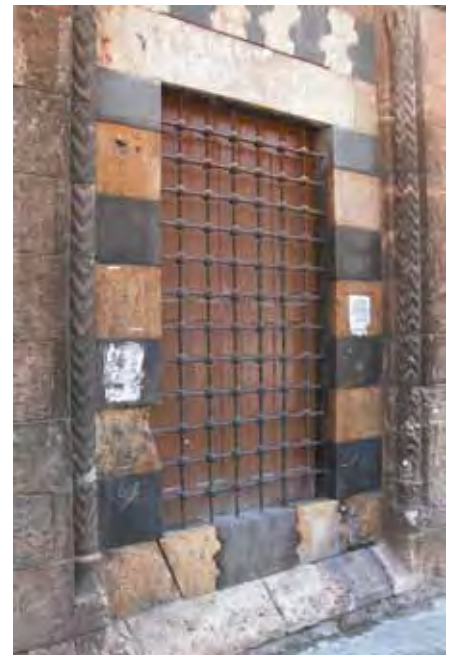
Figure 12 Al-Atrush Mosque, Aleppo, 1393ff: exterior window with ablaq masonry and marquetry marble
