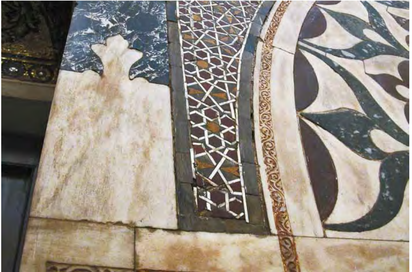
Figure 6 Zahiriyya Madrasa and Mausoleum of Sultan al-Zahir Baybars, 1277-81: interior with various types of mosaic in costly marbles and mother-of-pearl
