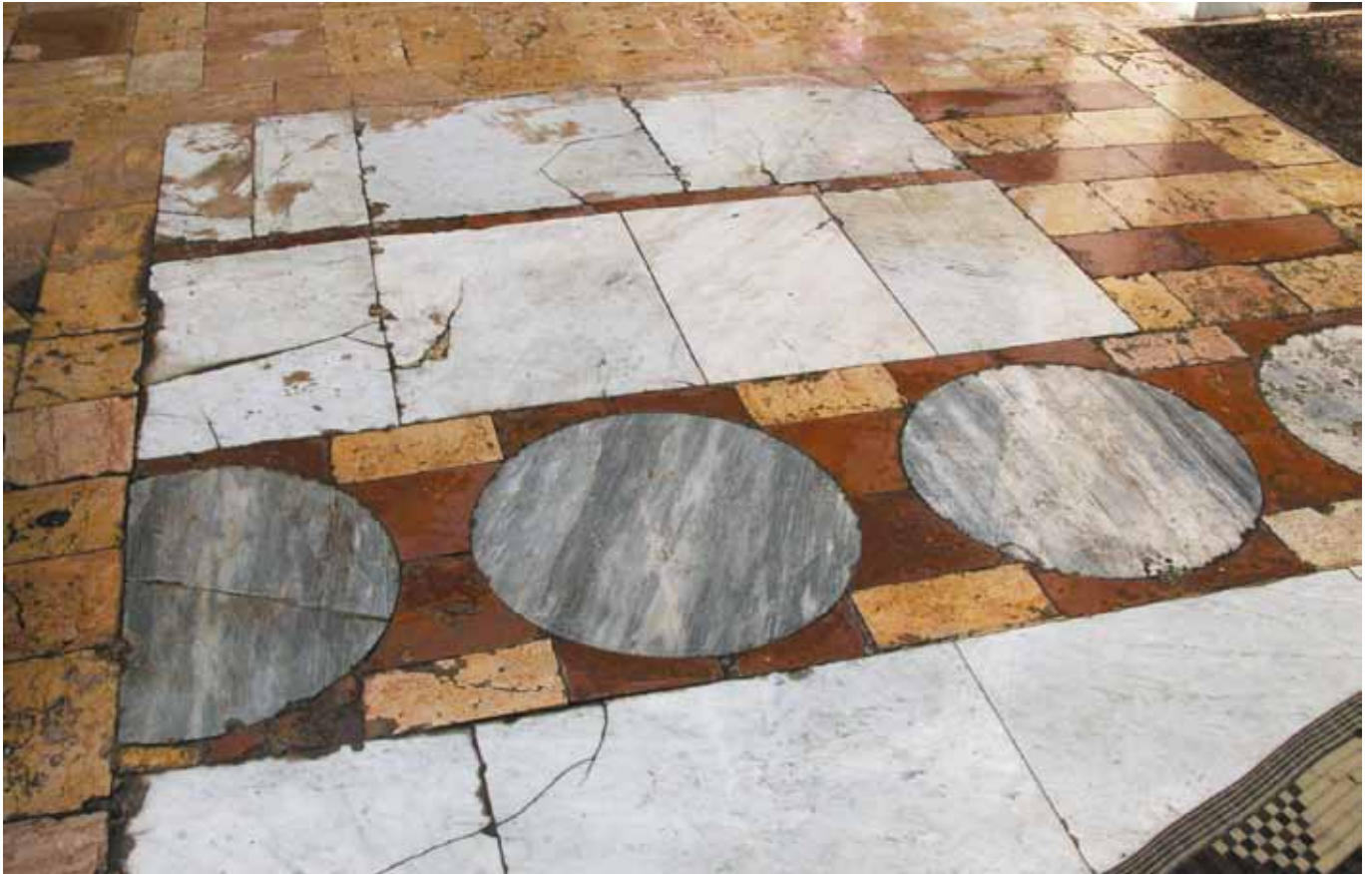
Figure 16 Damascus, Muhi al-Din ibn Al-Arabi complex, 1516, Damascus: courtyard mosaic floor, with roundels cut from antique columns
