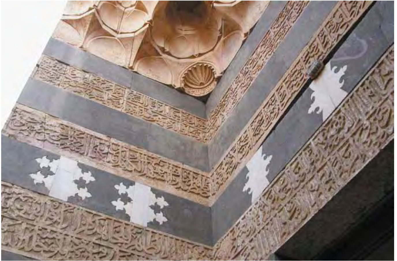
Figure 10 Zahiriyya Madrasa and Mausoleum of Sultan al-Zahir Baybars, 1277-81: exterior portal with marquetry marble decoration matching the intricacy of the limestone muqarnas
