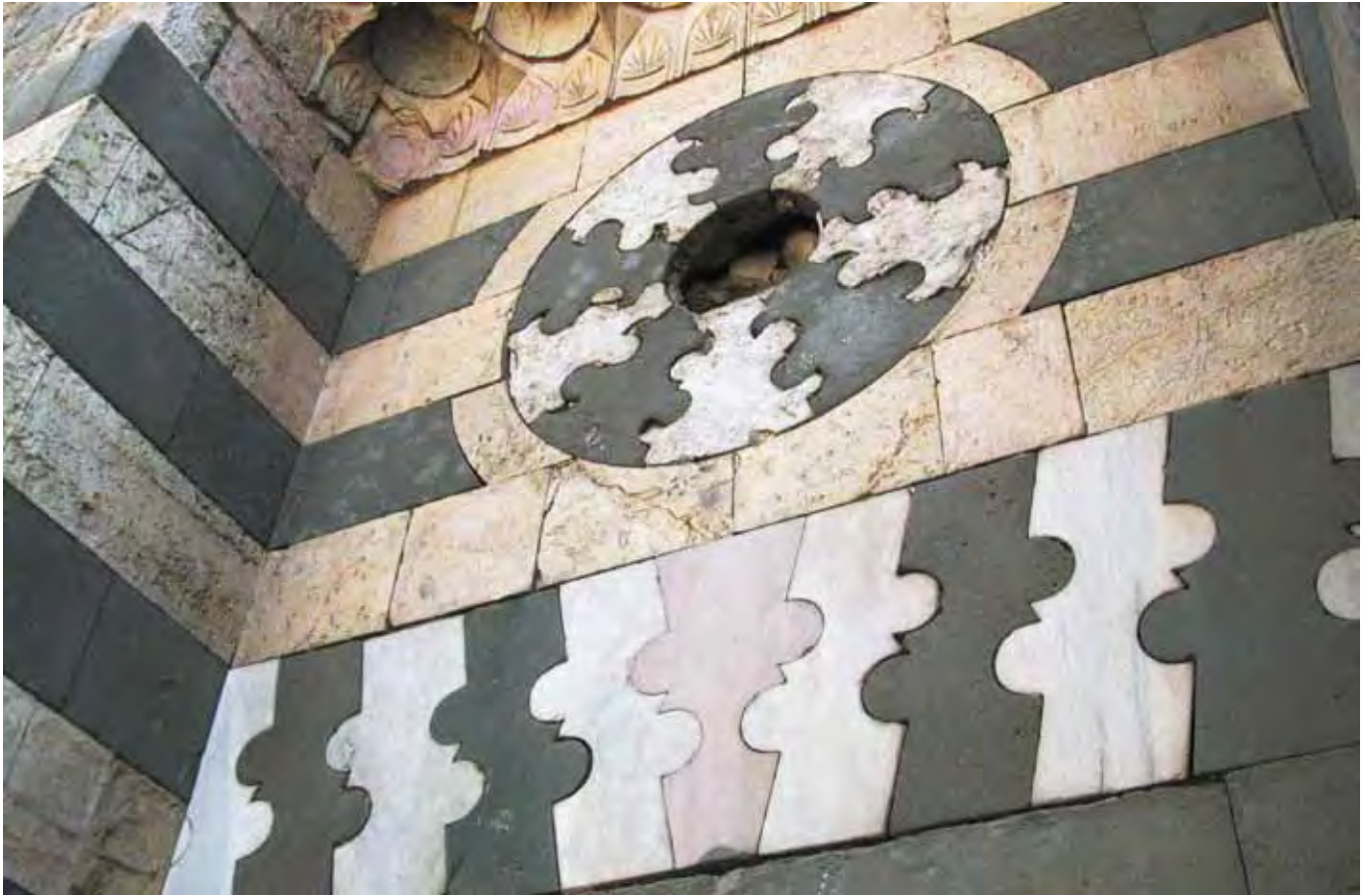
Figure 14 Mausoleum of Taynabak al-Hassani (or Al-Taynabbiya) 1395, Damascus: exterior portal with marquetry marble and other stones
