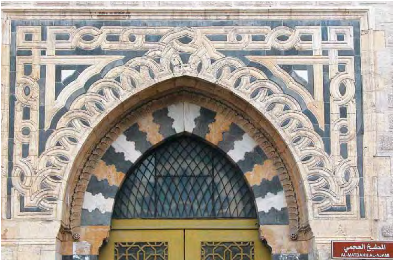
Figure 13 Matbakh Al-Ajami, Aleppo, early 13 th C: exterior portal with marquetry of marble and limestone
