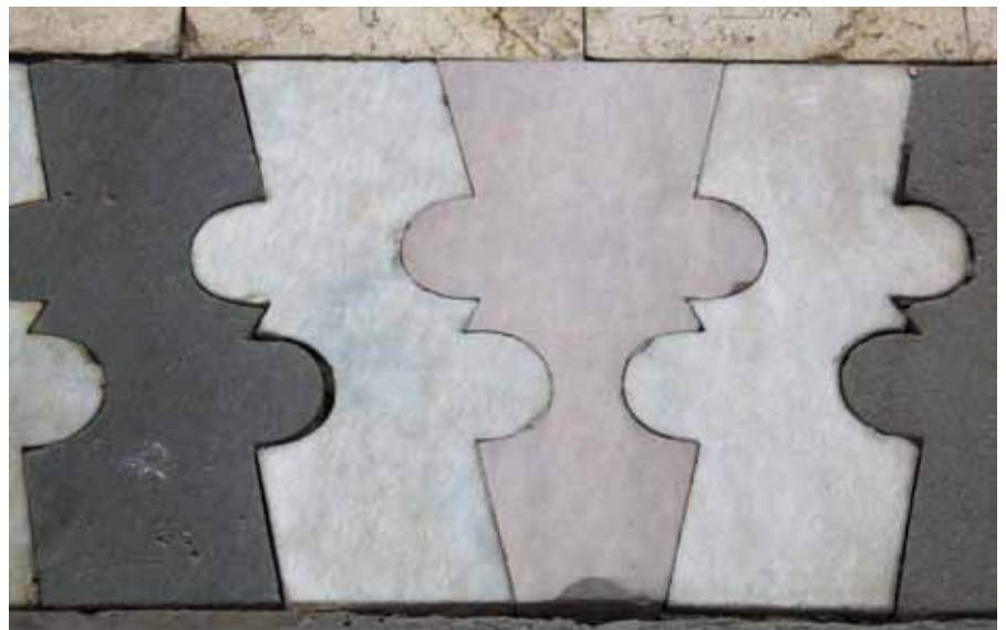
Figure 15 Mausoleum of Taynabak al-Hassani (or Al-Taynabbiya) 1395, Damascus: exterior portal with close-up of marquetry marble
