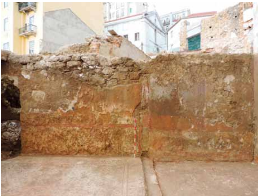
Figure 4 North wall painted plasters
