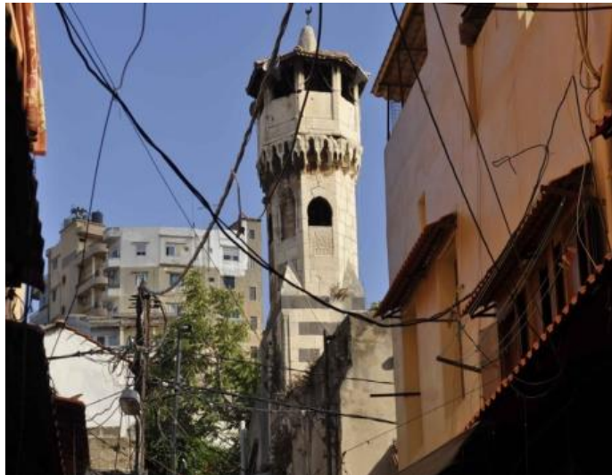
Figure 4. 13. Exterior of Al Tahan mosque (Hamid 2016)
