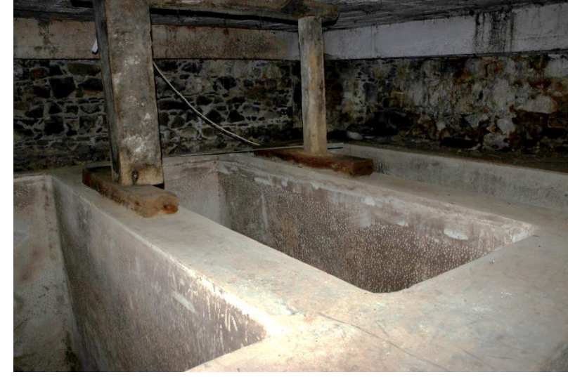
3) B01 BETONARME ZEYTİN HAVUZLARI
