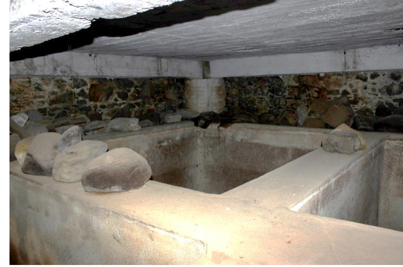
6) B01 BETONARME ZEYTİN HAVUZLARI
