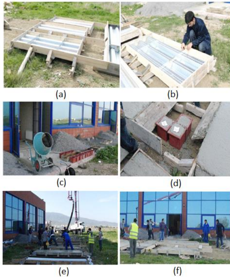
Figure 2.4. Installation of composite slabs (Başürücü 2013)
