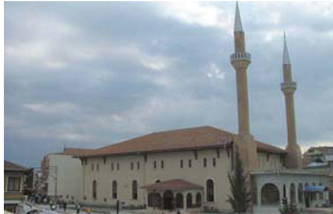
Fig. 13 Duzce Merkez mosque after retrofit (Duzcetanim 2008)
