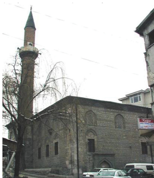
Fig. 7 Sarachane mosque and its undamaged minaret
