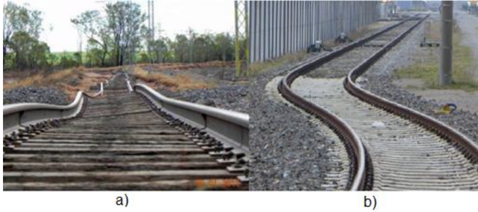
Şekil 2.53. a) Burkulmuř hat (Anonim, Twisted rail, 2021), b) S kurp (Anonim, Test and Validation Center in Wegberg-Wildenrath, 2022)
