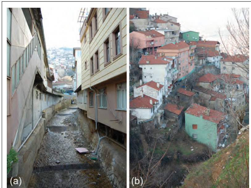
PHOTO 5A AND PHOTO 5B Examples of the existing problems regarding the stream
