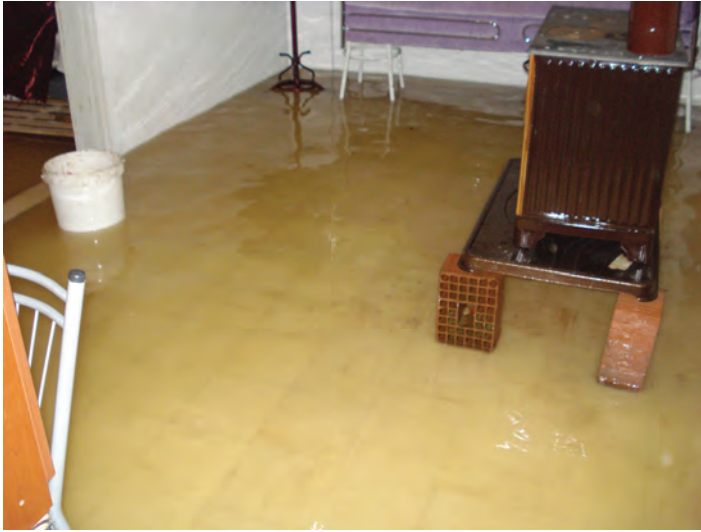
PHOTO 4 Affected house in Panayır
