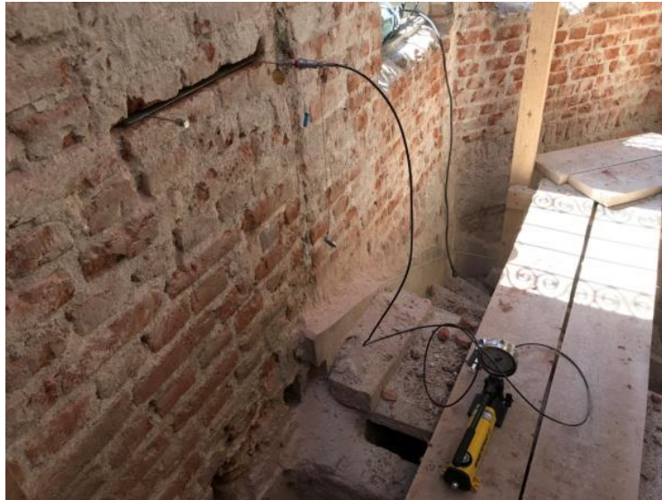
Figure 7. The mechanical tests: Single flat-jack test
