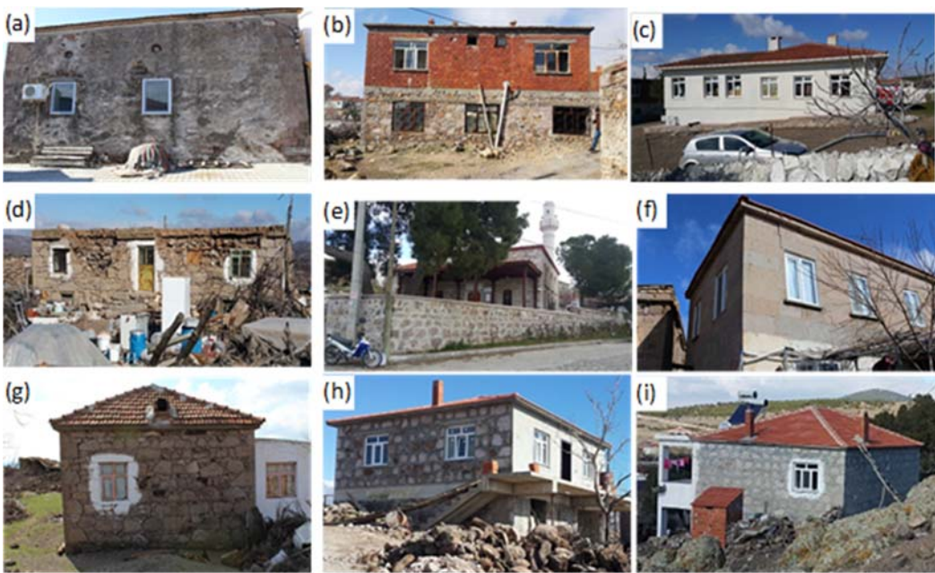
15 Figure 4: Existing building types in reconnaissance area: a) hatil dwelling b) stone and brick in cement mortar, c) engineered RC building d) hatil building with heavy roof, e) historical masonry with cut stone, f) cut stone without mortar, g) stone without mortar, h), i) stone in cement mortar with reinforced concrete.
