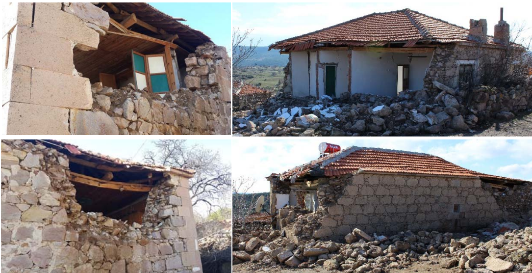
10 Figure 24: Out of plane failures due to improper wall thickness and/or height-length ratio
