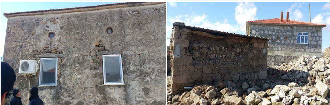
Figure 22: Examples of undamaged dwellings
