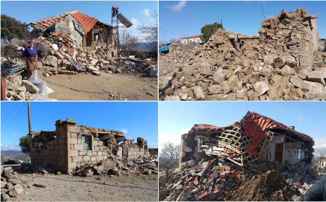
5 Figure 16: Examples of totally collapsed structures from Ayvacık, Çanakkale 2017 earthquake swarm
