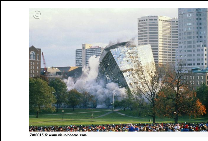
Figure 4.60 First positive example for damage
